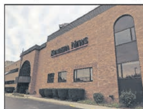
Starting Monday, the Kenosha News will no longer be located at the familiar 5800 Seventh Ave. building.
