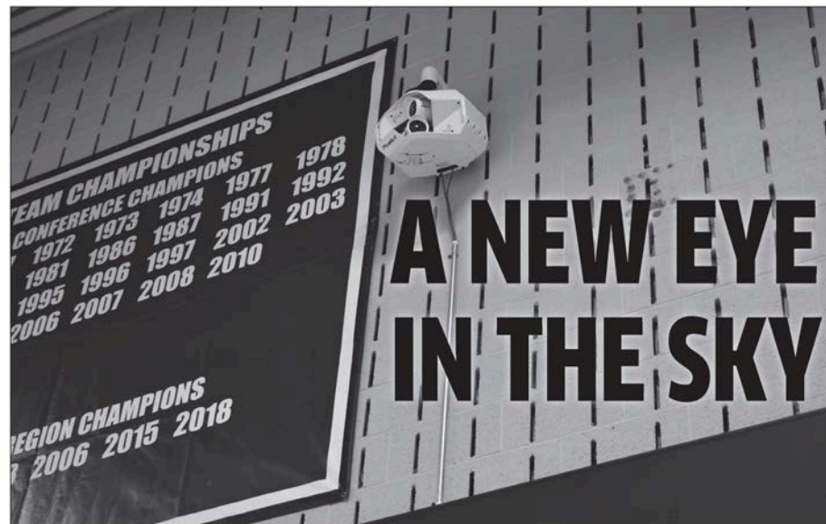
A new Pixellot Artificial Intelligence camera system has been installed in Redsten Gymnasium to help broadcast Madison College athletic events. Similar cameras have also been installed on the outdoor athletic fields.
