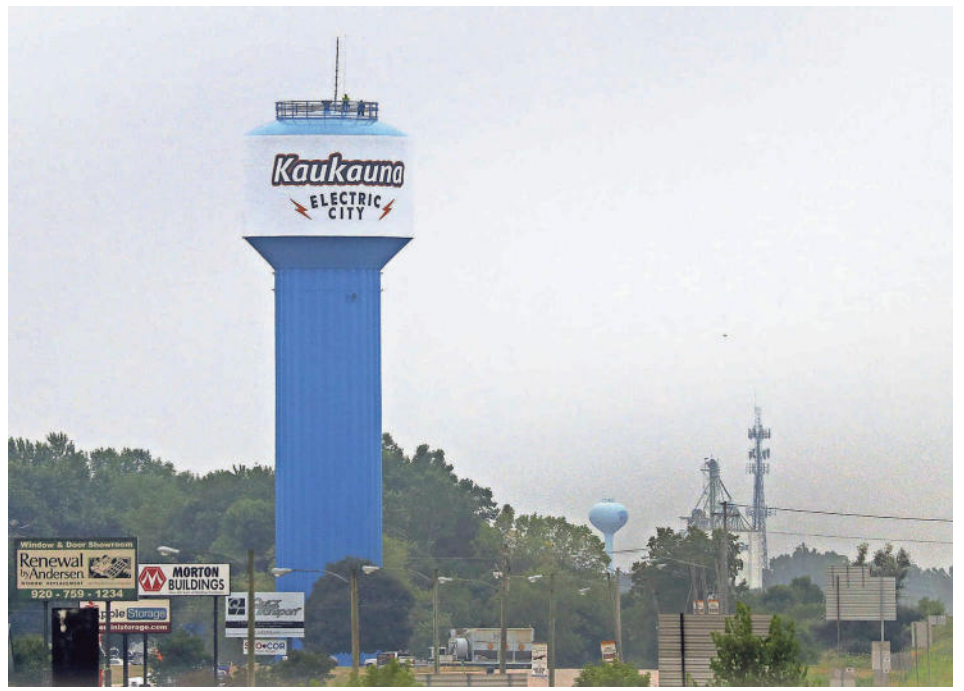
Water towers, like this one in Kaukauna along Interstate 41, maintain water pressure for distribution to customers. WM. GLASHEEN/USA TODAY NETWORK-WISCONSIN
