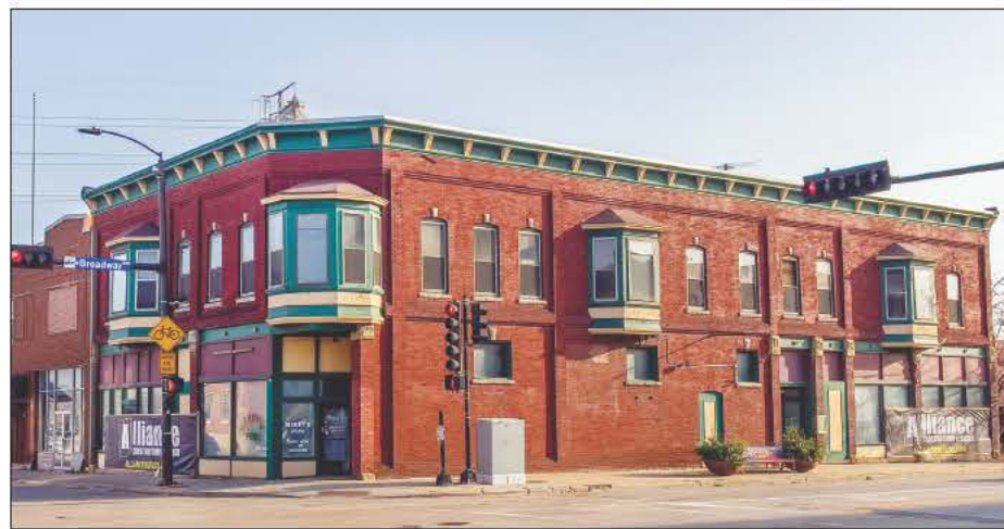
The three small saloon windows facing Broadway are considered critical to the historic integrity of the now-vacant building on the corner of Broadway and Dousman Street in downtown Green Bay. Daniel Kramer Photo
