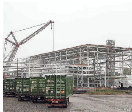
Construction on a new recycling facility is seen in progress.
