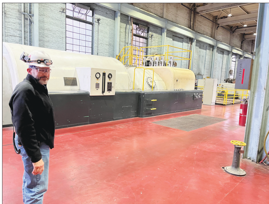
David Fulweber, Xcel Energy Bay Front Power Plant's general operations manager, next to one of the plant's two remaining and functional turbine-generators. (Peter J. Wasson/Staff photo)
