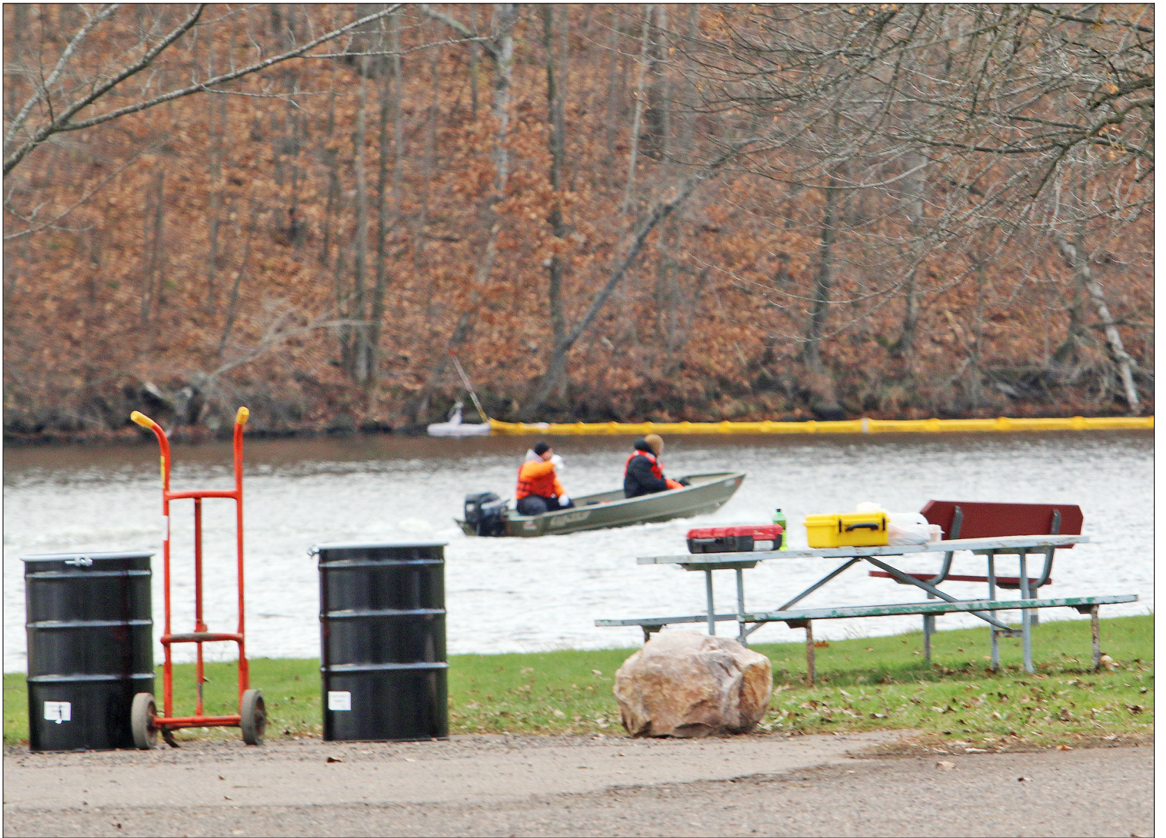
RIVER SPILL CLEANUP CONTINUES — Workers of an environmental and industrial services company head upstream in the Flambeau River on Saturday afternoon, using hundreds of feet of brightly colored yellow booms and barrels in an effort to contain a spill of turbine lubrication oil from the hydroelectric station at the Ladysmith Dam. The spill was initially reported as about 20 gallons, but later expanded to 175 gallons of the product labeled as non-hazardous. However, river residents reported to law enforcement seeing an oily sheen in the water and smell of gas in the air.
