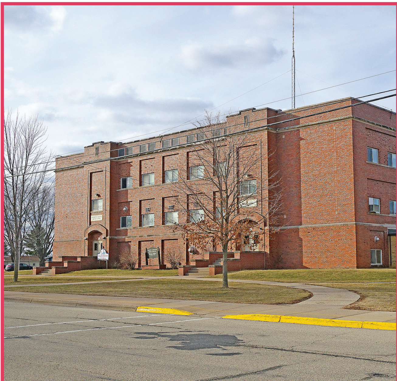
The sun is setting both literally and figuratively on the 1925 Lancaster Middle School Building, also known as the Winskill Annex. The Lancaster Community School District has stated they plan to tear the building down, and it may not standing on what would have been its 100th anniversary of its opening.
