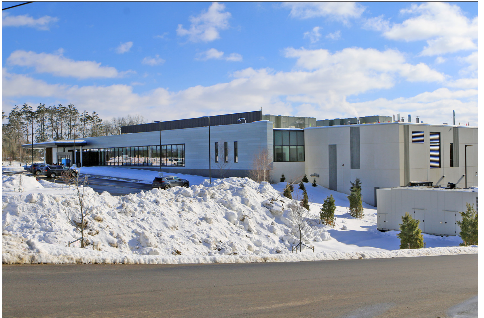
OPENING SOON — Marshfield Clinic Health Services officials are projecting its new medical center in Ladysmith will be fully open on March 13 after emergency and in-patient units are moved two days earlier. The facility features 75,000 square feet of departmental areas and 98,000 square feet of floor space combined on two levels. Clinic treatment rooms are in the upper level along the street, where the majority of people will enter. Hospital, emergency and extended stay rooms are on the lower level on the east side of the building. More pictures of the center's interior are in this week's Ladysmith News .
