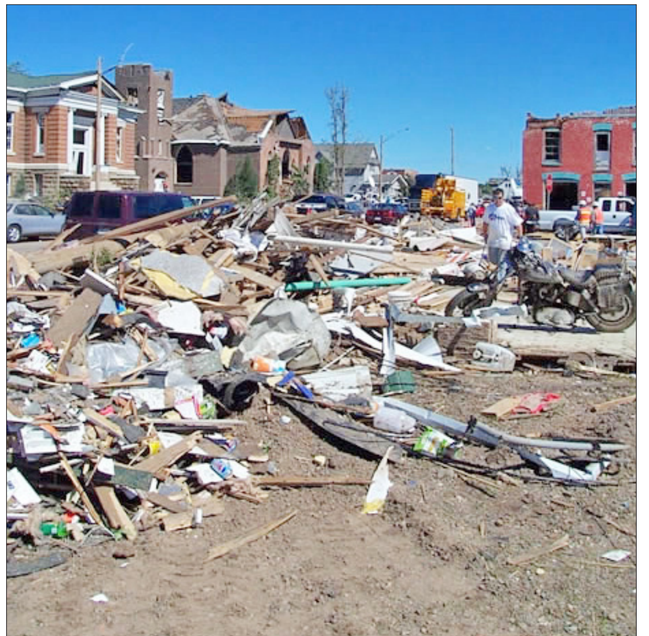
A REAL MESS — Tornado damage begins piling up along Lake Avenue as construction materials begin piling up for disposal. For about 30 minutes, the twister was in contact with the ground, raking a swath of devastation 15 miles long and 400 yards wide across central Rusk County. The funnel sucked back up near Ingram, and it was over.
