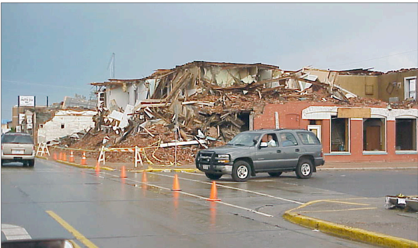
BUILDINGS LEVELED — Numerous buildings in Ladysmith were severely damaged or destroyed entirely by the severe tornado including this structure that had housed the former Enerson Ford dealership.
