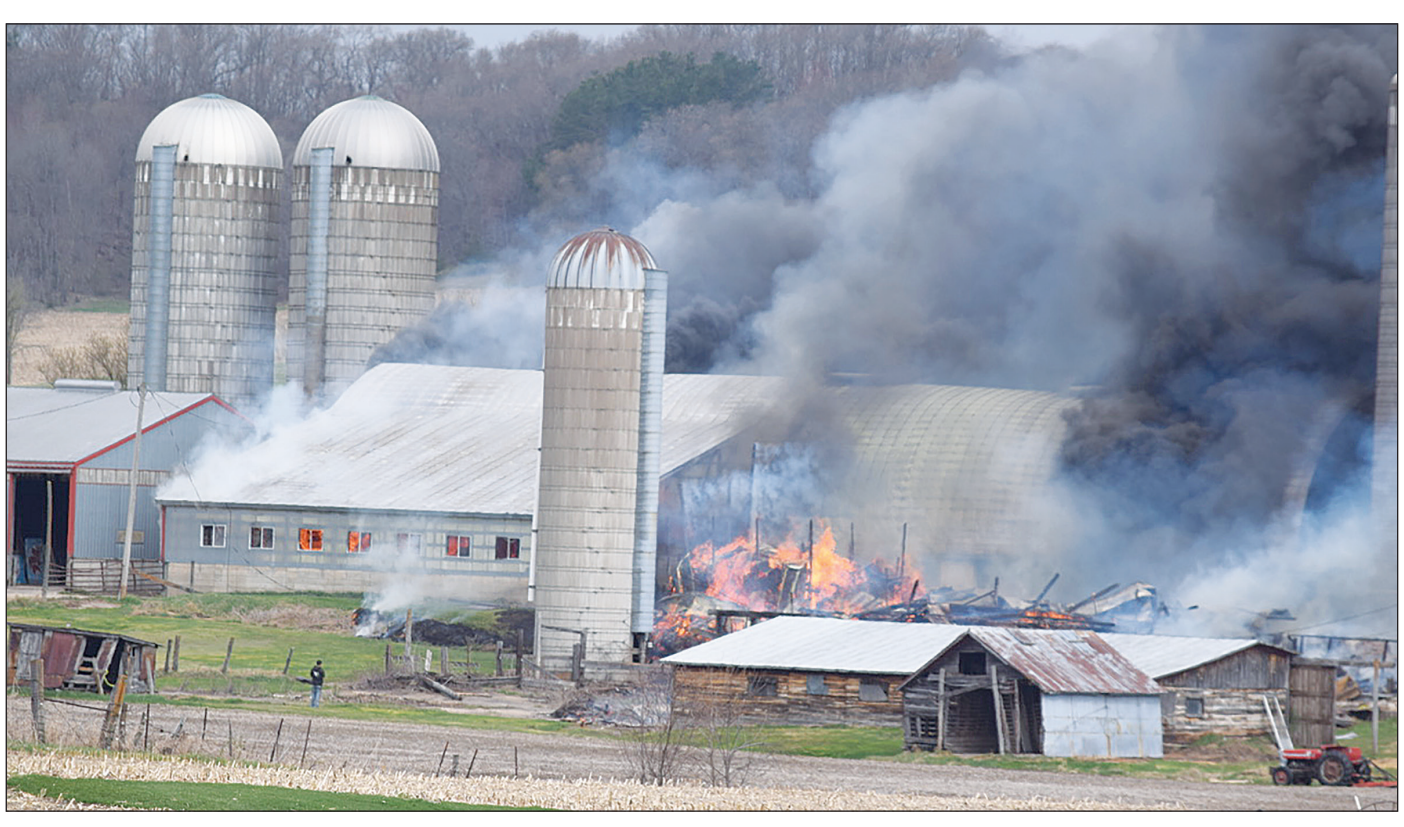
The Sparta Area Fire District responded to a large structure this (Thursday) morning at 9:45am. The fire was a barn/shed located at 8167 County Highway BC in Sparta. More information on the fire will be in Mondays paper. Herald photo by Kyle Evans.
