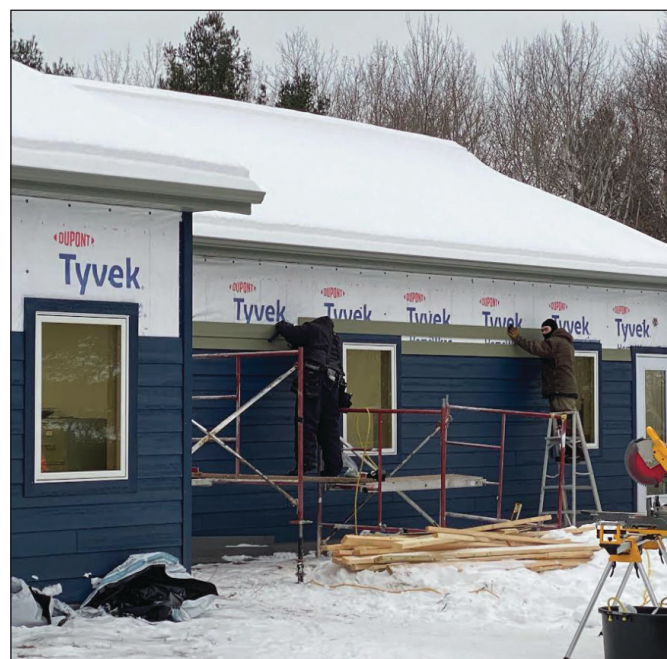
The former Northern Edge Sports Bar and Fore'n Aft restaurant has gradually been remodeled and updated for the move. (Photo contributed by Big Top Chautauqua)
