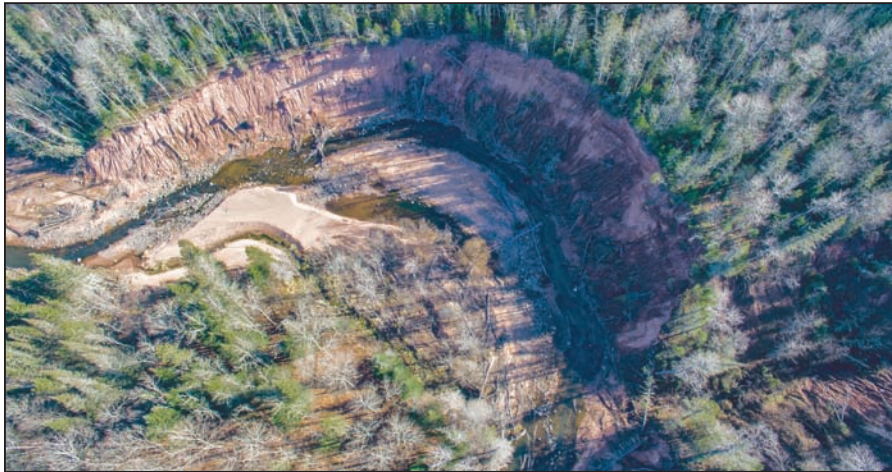
An aerial photo makes erosion on North Fish Creek apparent even top untrained eyes. With every storm, more of the bluff erodes and flows into the bay. (Contributed photo by Bob Gross.)
