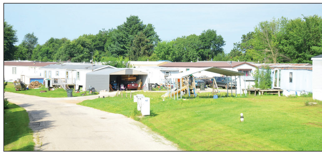
Ageing trailers with little room to spare make Cozy Acres feel crowded and cluttered. A public play structure shows signs of age and misuse.
