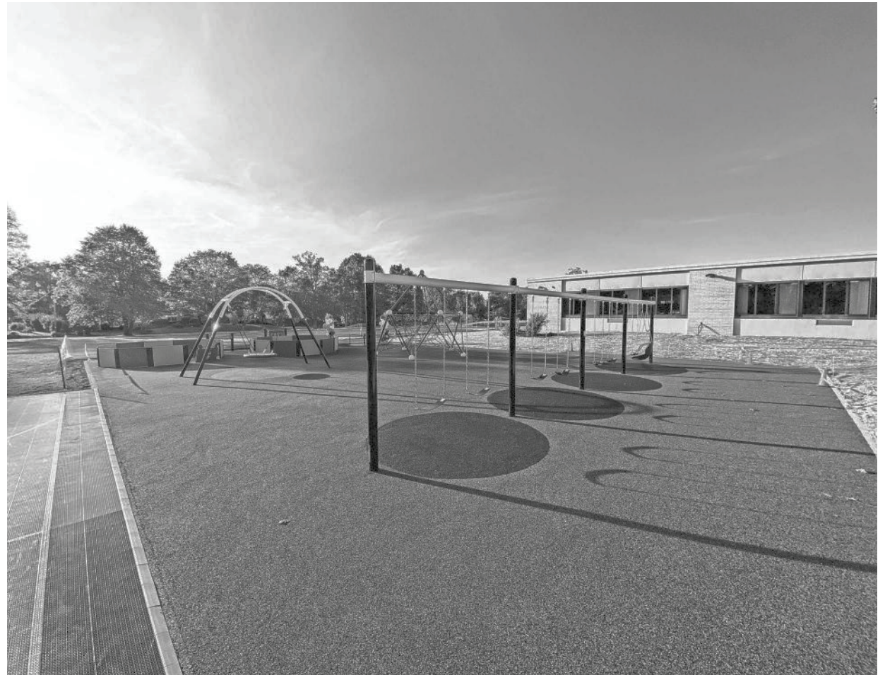
The Fox Point-Bayside Educational Foundation raised $210,000 over a two-year campaign to establish the first ADA-accessible playgrounds in the community. The playgrounds are at both Stormonth Elementary School and Bayside Middle School. SUBMITTED
