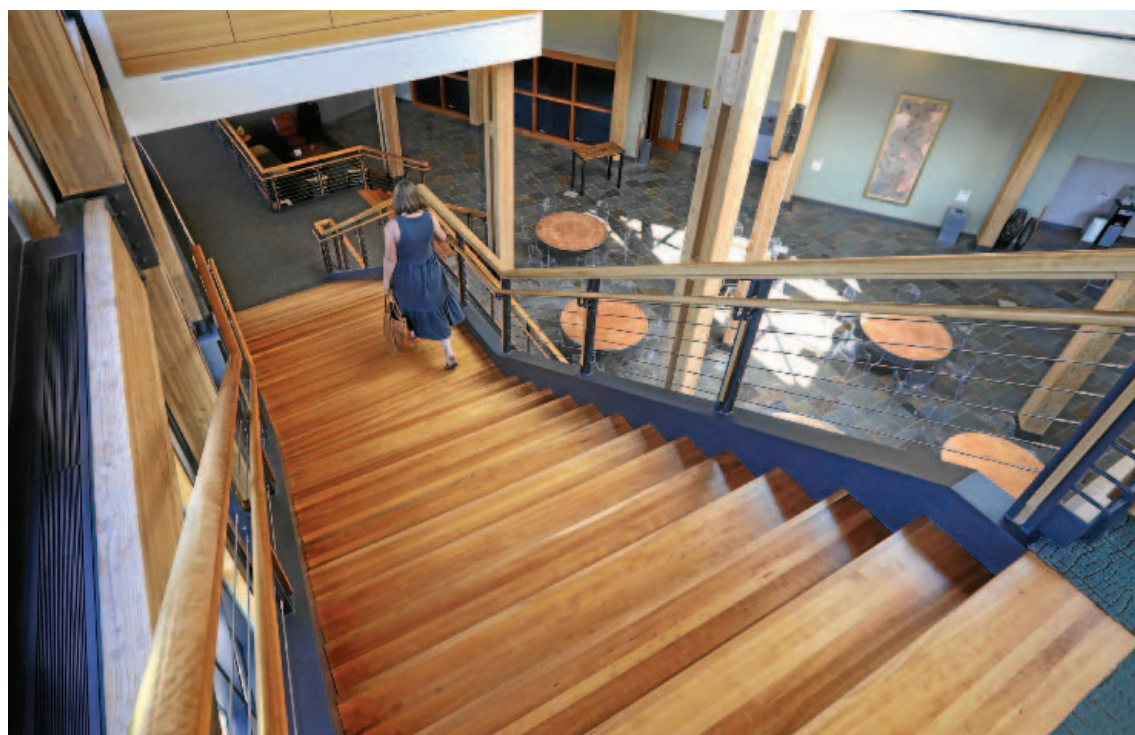
The stairs at Promega's Feynman Center are made from walnut trees harvested on the company's property in Fitchburg, which architect David Rousseau said was an effort to honor the trees.
