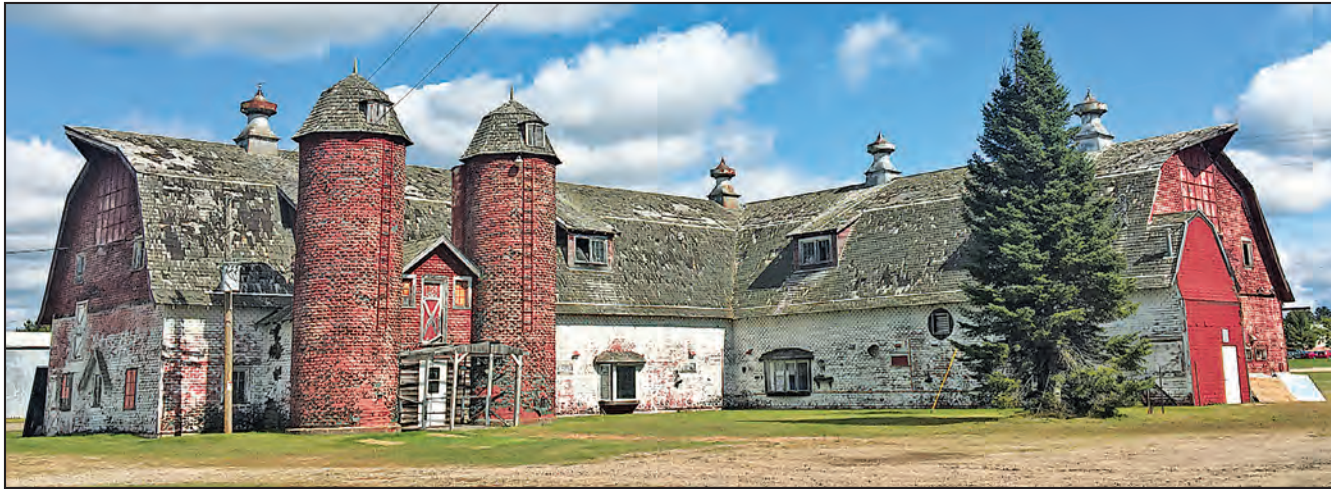
Still a distinctive sight on Eagle River's North Woods skyline, the circa-1925 M&R Dairy Farm barn complex was repurposed in 1962 as Big Barn Shops, housing 15 shops, restaurants and a bar in the 1960s-'80s. A third barn wing to the south, which
