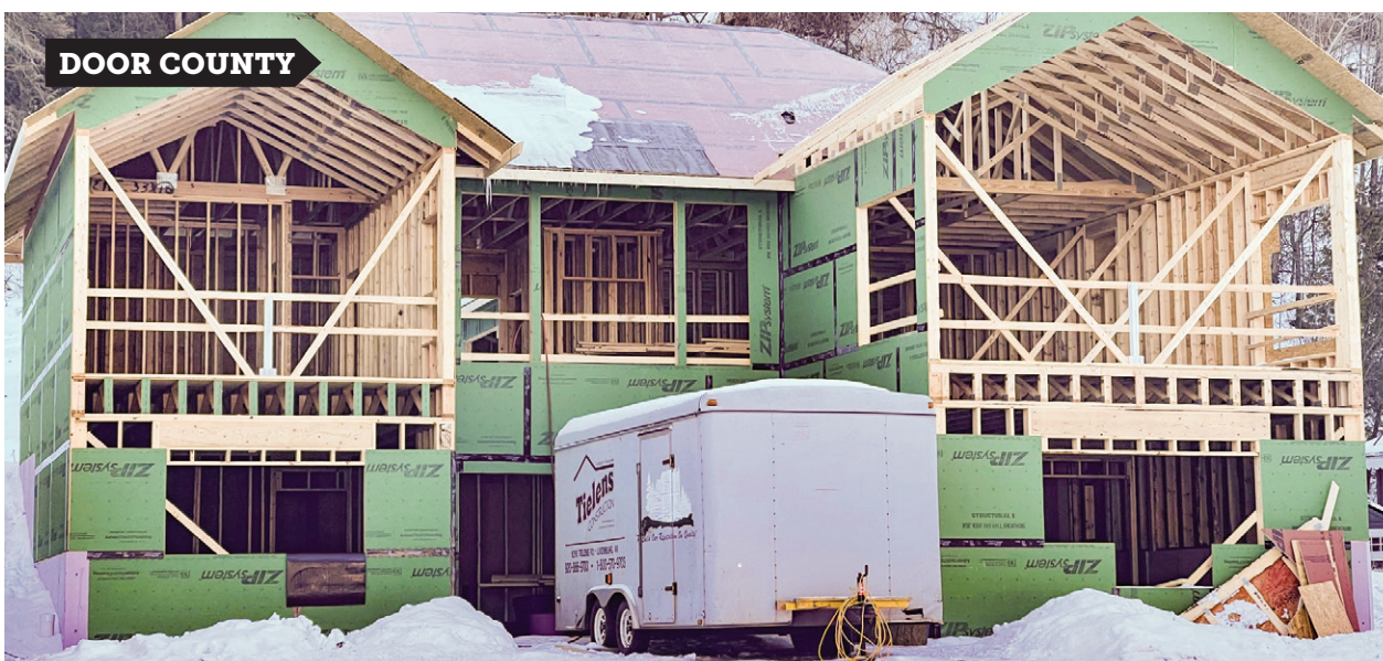
Existing housing stock sold quickly once it was on the market during the past two years, causing many buyers to scoop up land and go the route of building their own, such as this home under construction on Bay Shore Drive in Sevastopol. Photo by D.A. Fitzgerald.
