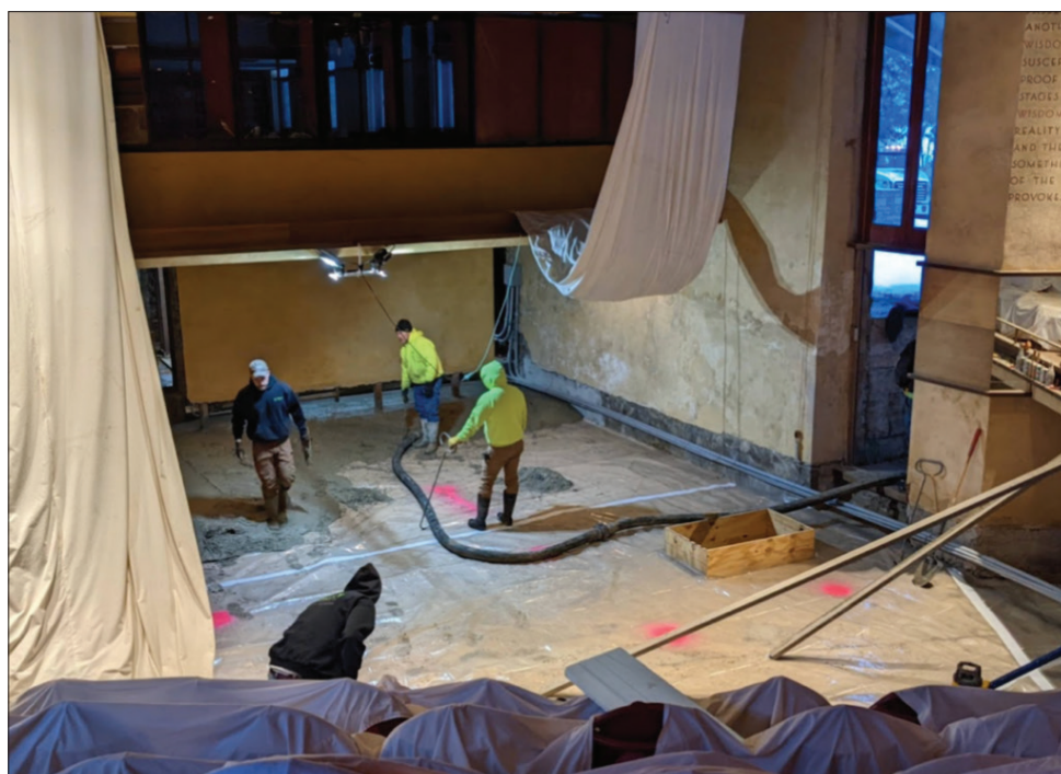
Photo contributed by the Taliesin Preservation Concrete pouring in the Hillside Theater.
