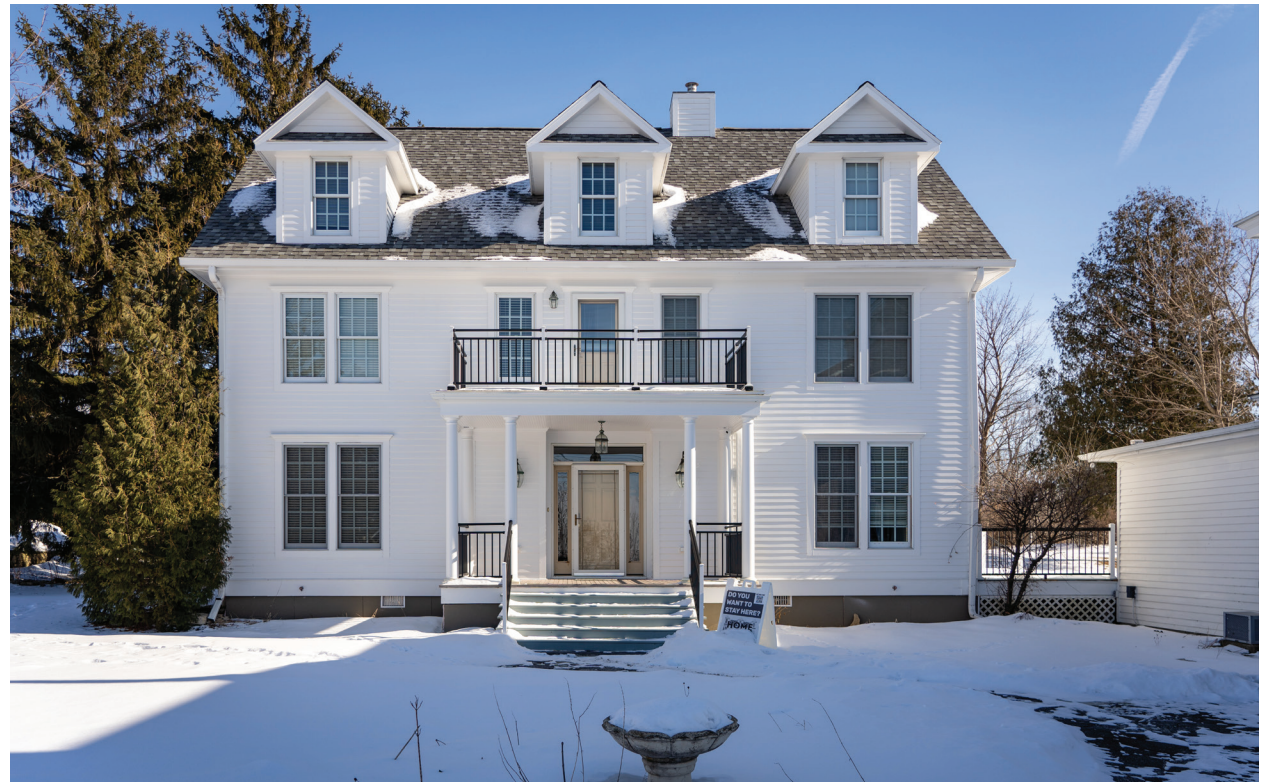
The former home of Doc Eames will eventually become a bed-and-breakfast. The building was moved to the property from Eames Farms on the hill east of the village in the 1990s. Photo by Rachel Lukas.
