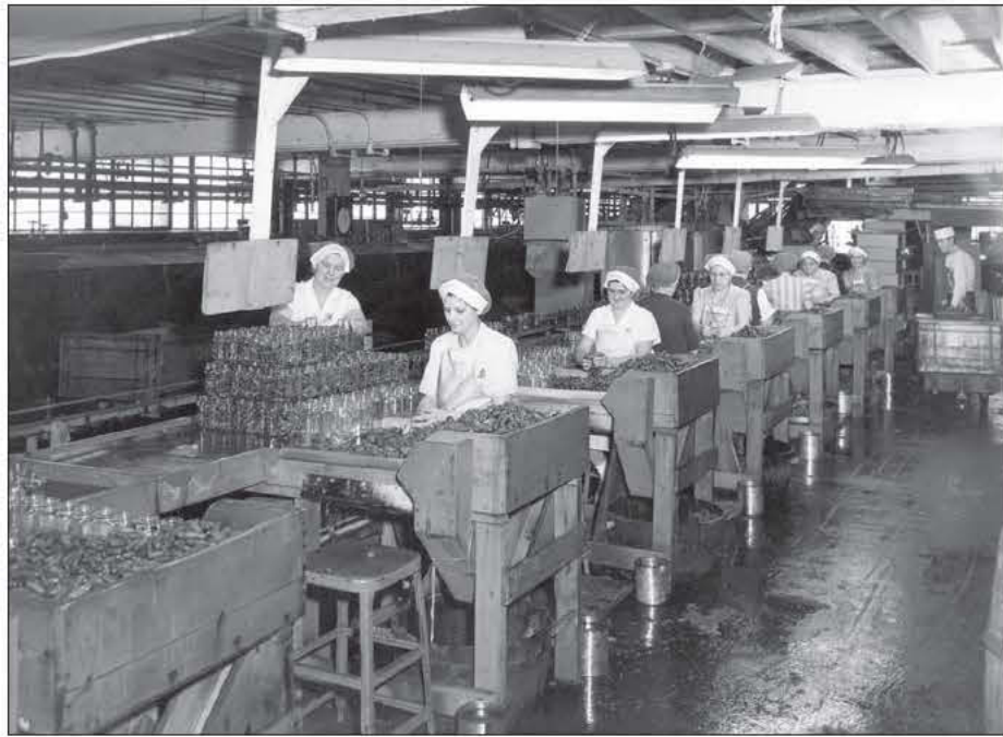
Workers fill pickle jars at the former Balza Pickle Factory in Howard, which later became Stokely Canning. The building is set for demolition beginning this month. Submitted Photo
