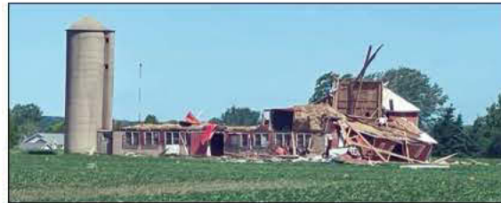
A confirmed EF-1 tornado destroyed structures throughout Seymour.
