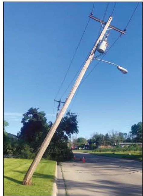
Damaged power line poles on Lenwood Avenue in Howard.
