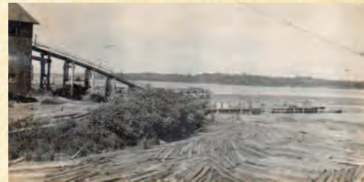
Logs are slid into the lake to be run 50 miles downstream on Red Cedar River to Menomonie.
